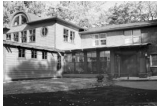
Thor Badendyck's first-floor addition to his parents' home features a covered entryway, sunroom-style vestibule, and sky-lit art studio.
